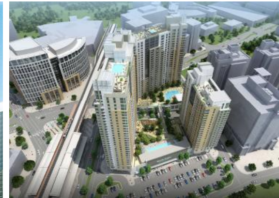
Hoffman Town Center (Alexandria, VA) 1242 Multifamily Units + 46K SF Retail (residential towers) and 670K SF Office and 29K SF Retail (National Science Foundation Headquarters)
